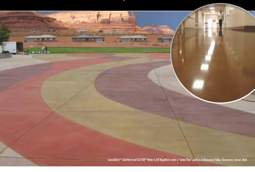
Consolideck® ColorHard is a premeasured color concentrate. Simply mix 4 ounces with 1 gallon of Consolideck® LS® lithium-silicate hardener/densifier, or LS/CS® for a ready-to-use color hardener.
